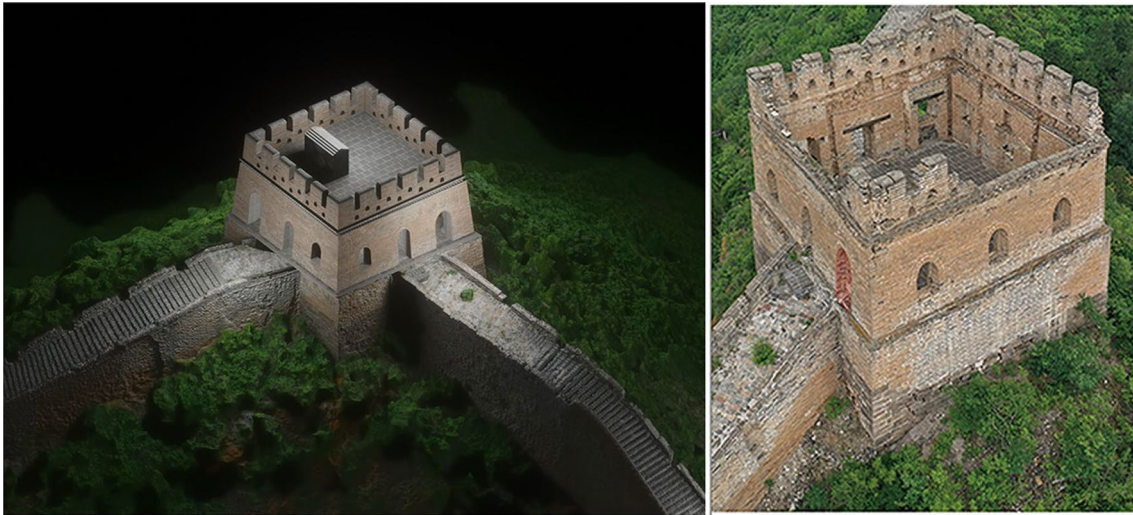
Three-dimensional model of the current condition and restoration of the hollow watch tower
