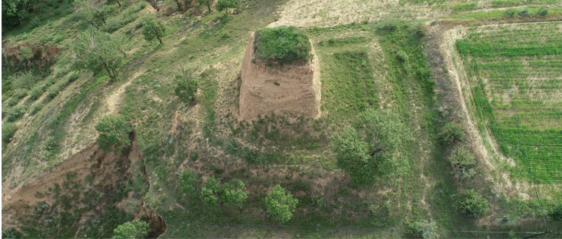
Three-dimensional point cloud model of the current condition and restoration of the beacon tower
